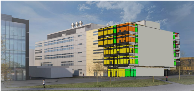
← BCE Dynamics: Building simulation to assess the air conditioning requirements of rooms at the University of Lübeck. (Image: GM.SH, Grawunder Design)
